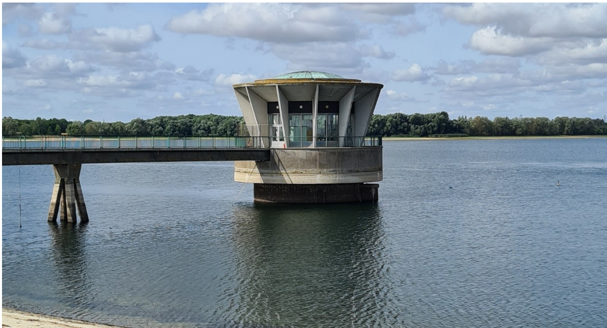
Image 2.6: Example of an outlet tower
